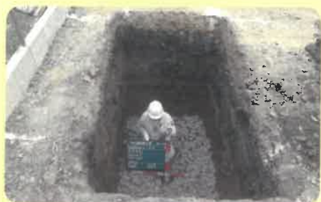
No.3 地業工事[割栗地業工事]
